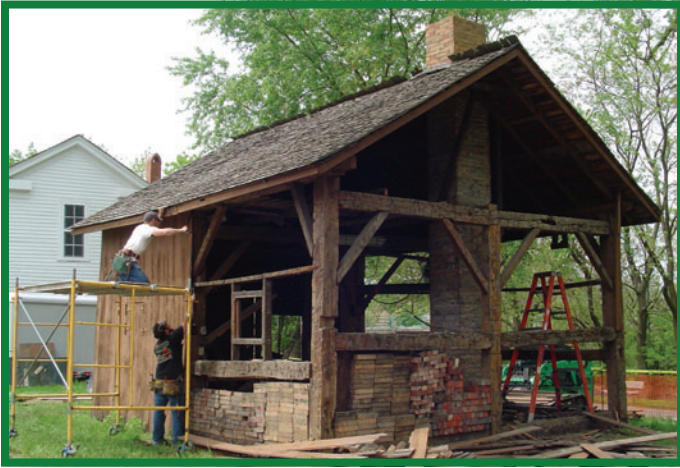
Above: Blacksmith's Shop dismantled for salvaged materials.
