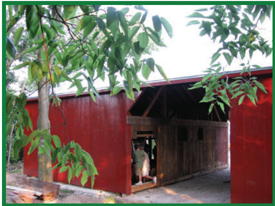
Above: Gindler Barn restored, July 2008.
