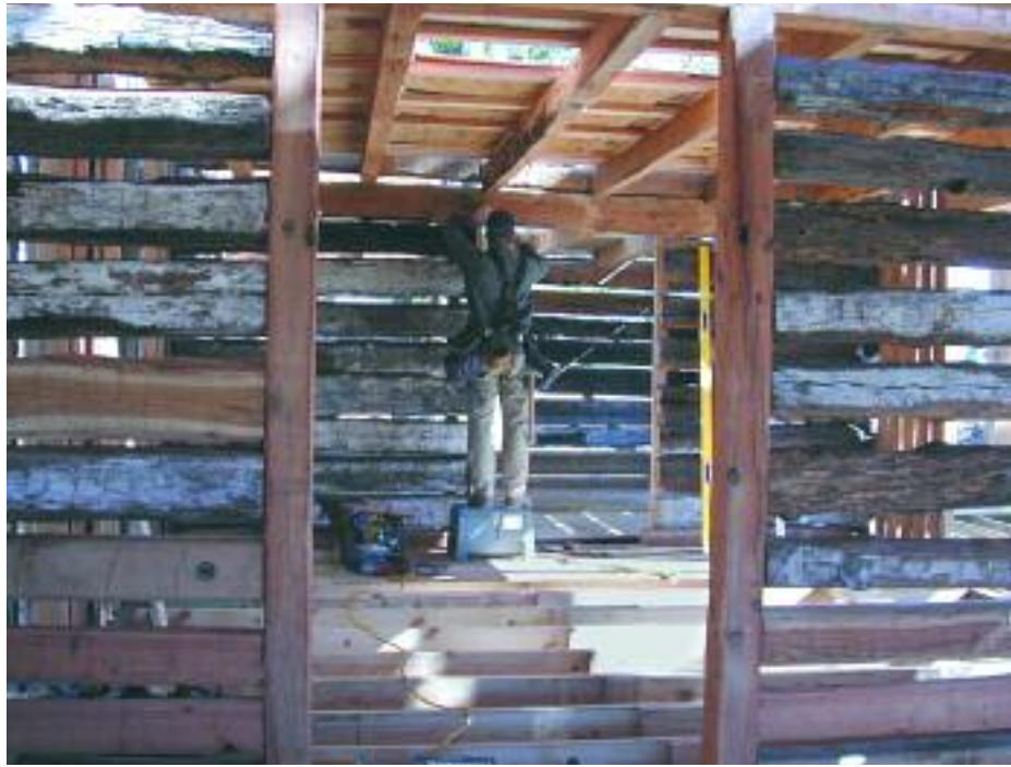
Fig. 5. Isaac McCoy at work on a plate log. Log walls are a mix of old and new.
