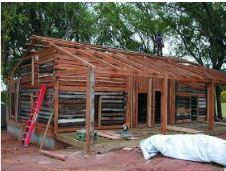
Figs. 2–3. Front and back walls show mix of horizontal chinker and a kind of stave construction. Concrete foundation and pressure-treated deck framing concede to modernity. On the roof, left photo, Rick Collins (l.) and Adrienne Walker; right photo, Isaac McCoy (l.) and Scott Russell.
