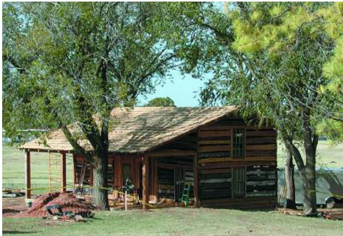
Fig. 6. Relocated and restored cabin reposes among American elms in Shawnee, Oklahoma.
