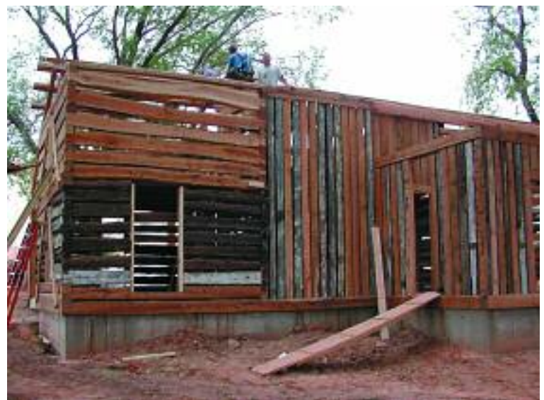
Figs. 2–3. Front and back walls show mix of horizontal chinker and a kind of stave construction. Concrete foundation and pressure-treated deck framing concede to modernity. On the roof, left photo, Rick Collins (l.) and Adrienne Walker; right photo, Isaac McCoy (l.) and Scott Russell.
