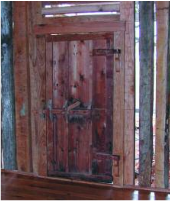
Fig. 4. Plank door swings on wooden pintle hinges.
