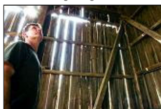
Rick Collins from Trillium Dell Timberworks examines the structural integrity and likes the high quality workmanship including the angled cross beams supporting the corner of the barn.
